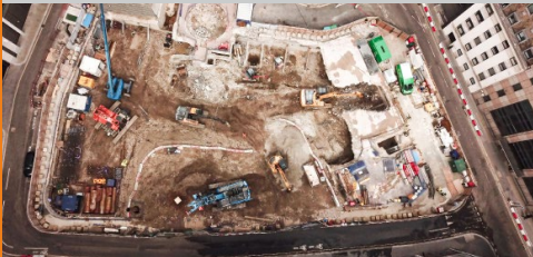
65 Crutched Friars (£820k): Downwell Enabling's first project for McAleer & Rushe involved substructure breakout and pile enablement works near Fenchurch Street station in the City of London.
