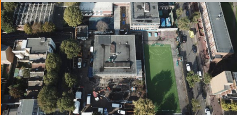
Bermondsey Campus (£2.95m): Demolition and ground remediation of school buildings, sports hall, and studios were completed in two phases to enable redevelopment into residential, commercial, retail, and public spaces.
