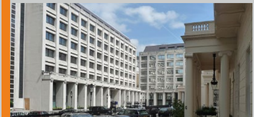
20-24 Carlton House Terrace (£30m): The Carlton House project in Westminster involved complex cut-and-carve demolition through a live car park, extensive temporary works across 15 floors, façade removal, and vertical cutting to enable construction of three additional cores.
