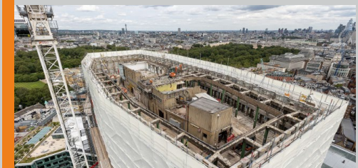
Portland House Refurb (£40m): At the 30-storey Portland House near Buckingham Palace, I delivered demolition enabling works including basement strip-out, decladding, lift removals, and preparation for crown demolition.
