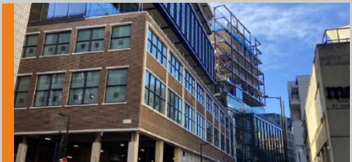
Timber Square RC New Build (£30m): At 25 Lavington Street, I led demolition and groundworks for the Timber Square development before being seconded as Project Manager to Swantest.
